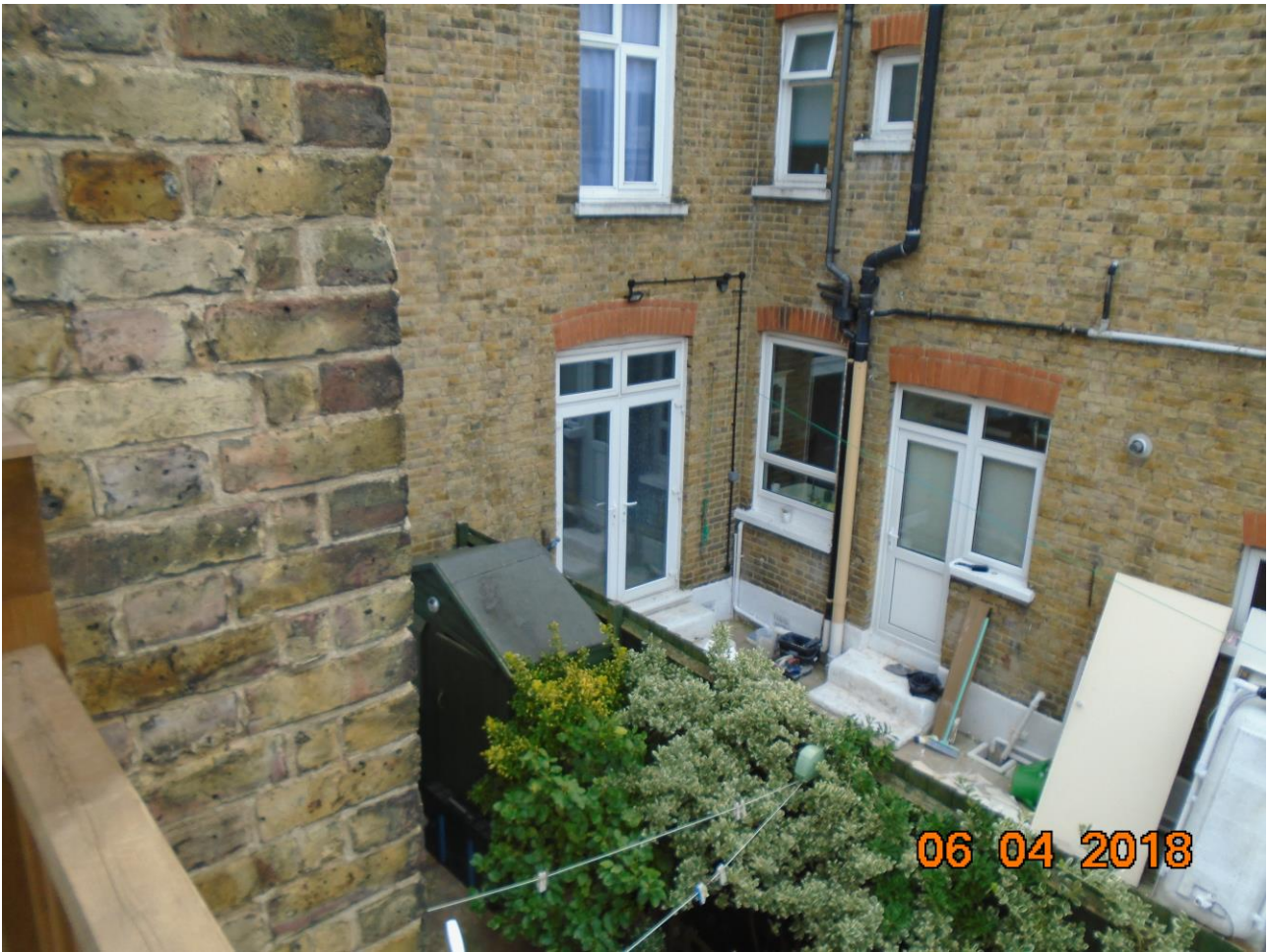
View to south from platform
